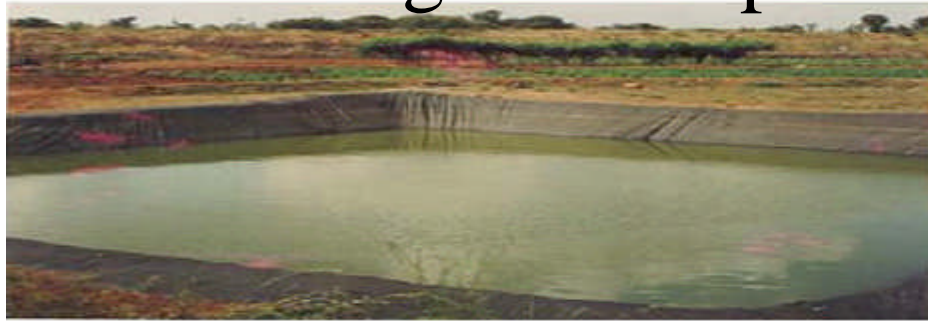
A farm pond lined with containment liner to control seepage
